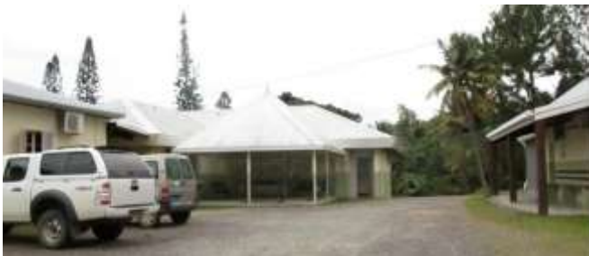
Photo: Health center, Pouebo, New Caledonia.
